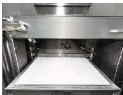
02 HEPA Filter Replacement
